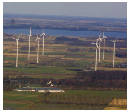
Windpark Damme, Borringhausen
